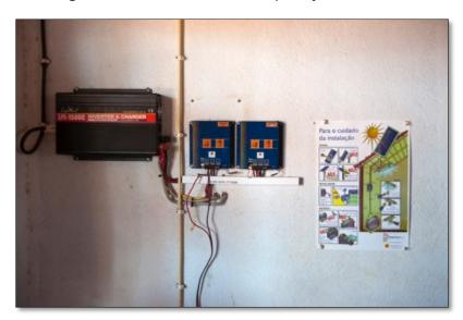
Photo 9: Image of a solar power system for refrigeration in the Clinic,
