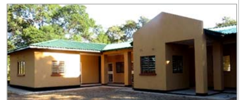
The Sioma Ngwezi main office complex
